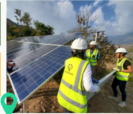
Installing 6kw of solar microgrids in a rural village
