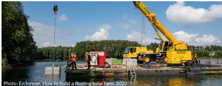
Photo: Enformer. How to build a floating solar farm. 2022
