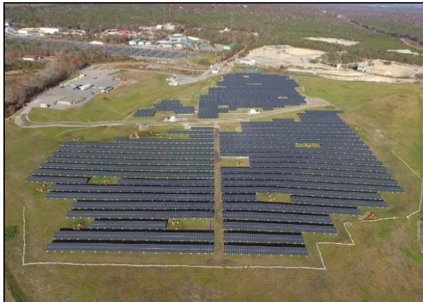
Example of our Landfill Solar Development
