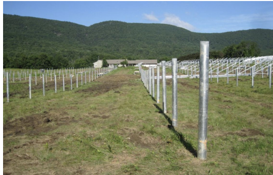
High Foundation Cost
