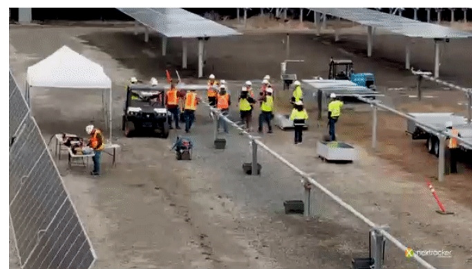
Installing PV Panels
