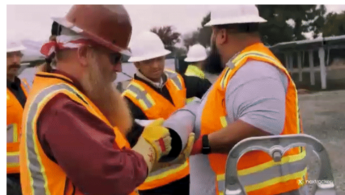
Installing Torque Tubes
