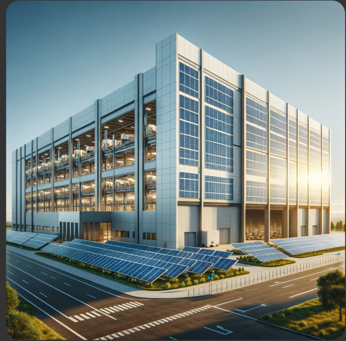
Solar Manufacturing First Solar
