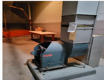
Figure 1: Existing AHU
