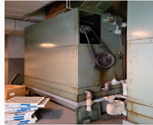
Figure 1: Existing AHU
