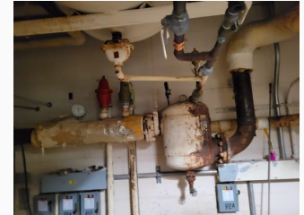
Figure 2: Existing Condition of bare piping
