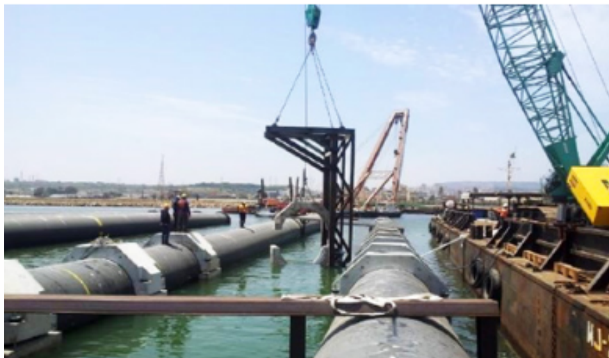
Figure 8. Concrete collars on a 2.5m water intake pipeline,
