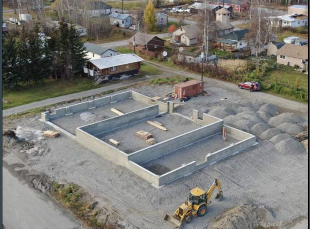
City of Nenana Biomass Plant foundation (2022)
