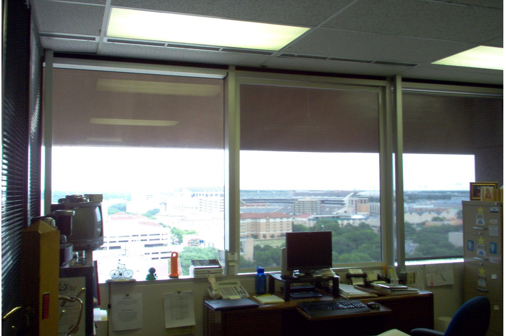
Texas Conservation Commission Building – AUSTIN, TEXAS Left Window – No Inflector Radiant Barrier Window Insulator
