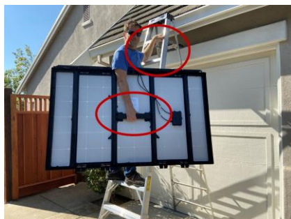
Carrying handle on backside of PV module
