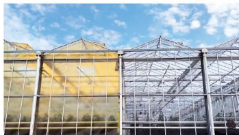
UbiGro film retrofit in a greenhouse
