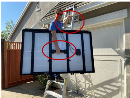
Carrying handle on backside of PV module
